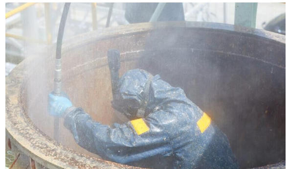
▲濃縮管超高压洗浄
