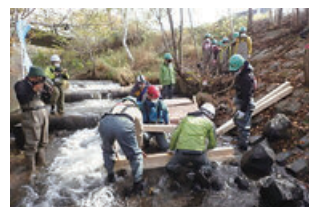
Okhotsk Fish Conservation Society • Installing fish ladders for salmon
